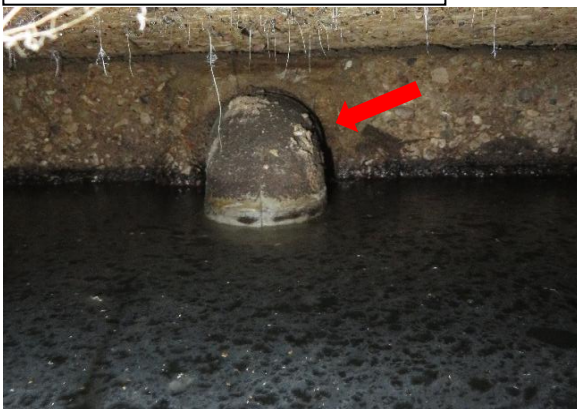
No effluent filter at outlet
