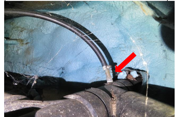
Water filter discharge to septic
