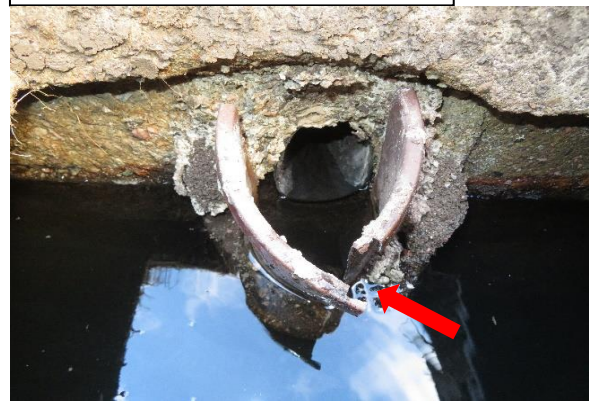
No effluent filter at damaged outlet
