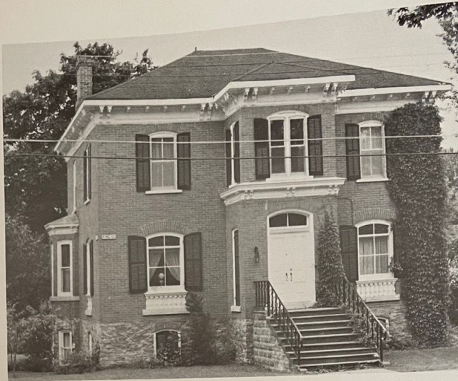
Oblique view: Youmans/Paul-Duddy House at King and Bowery. Here again is the characteristic 'Country' vestibule in the two-storey version.
