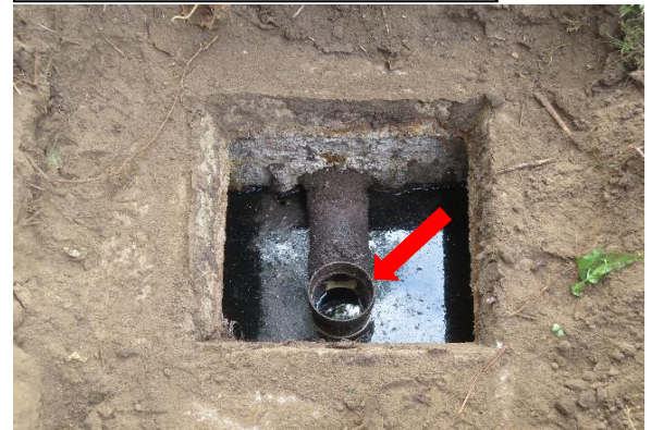
No effluent filter at outlet
