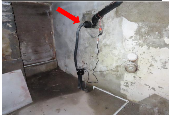
Sump pump discharge to septic
