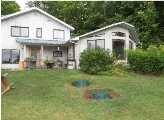
General tank location
