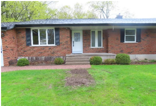
General tank location
