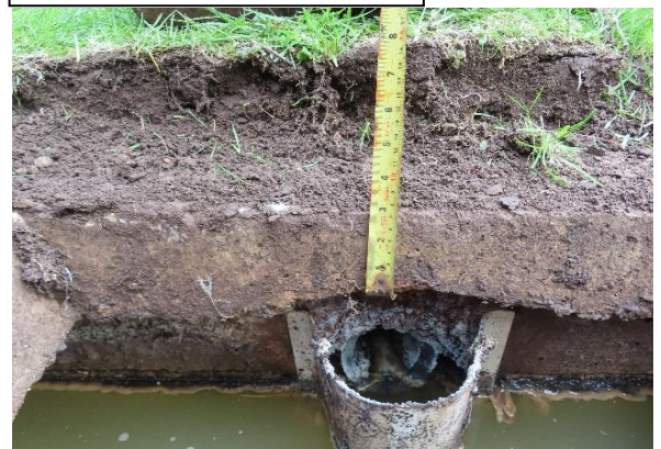
Thickness of concrete at outlet
