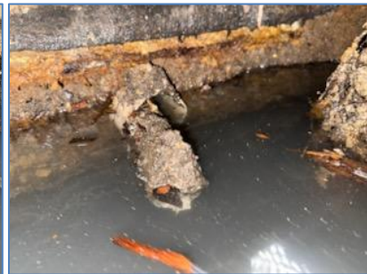
Fig. 6 – Liquid Flowing out of Forcemain
