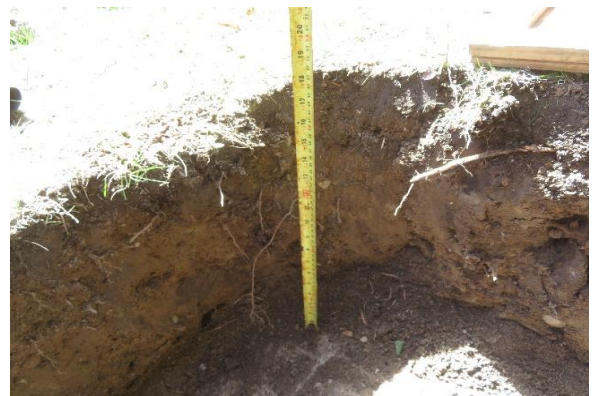
Depth to top of tank
