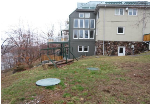
General tank location
