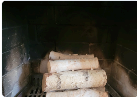
Main floor firebox interior — light sooting on refractory firebrick, normal use condition
