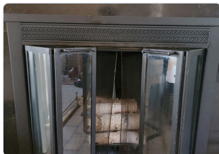
Main floor fireplace — bi-fold glass doors and metal mesh curtain in place
