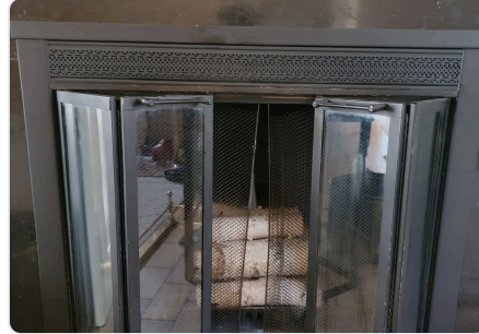
Main floor masonry fireplace close-up — bi-fold glass doors, metal mesh curtain, refractory firebox
