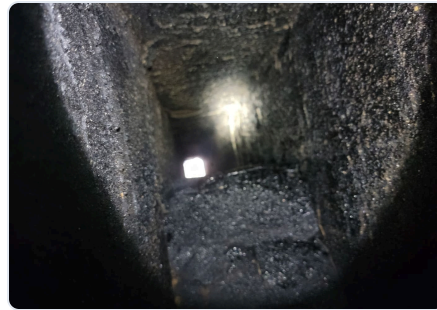
Main floor flue interior — low creosote level, flue open and unobstructed
