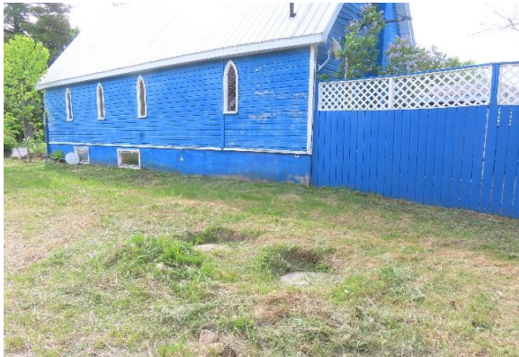
General tank location
