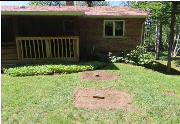
General tank location
